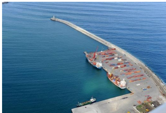
Figure 3. Container terminal of Praia da Vitória port.
